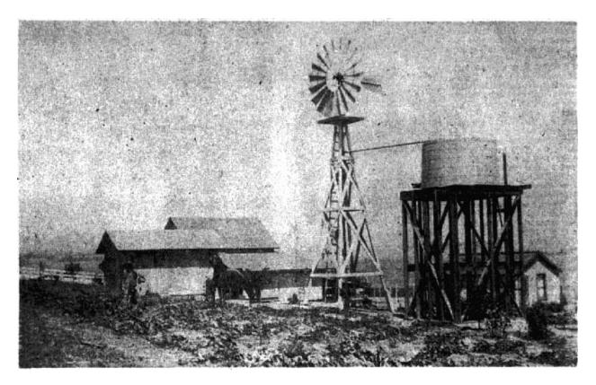
The Whitaker Ranch farm house, today the site of a Texaco gas station at Bundy and National. Windmill-powered water wells and gravity-feed water tanks were common in Ballona Valley in the late 1800s and early 1900s.
