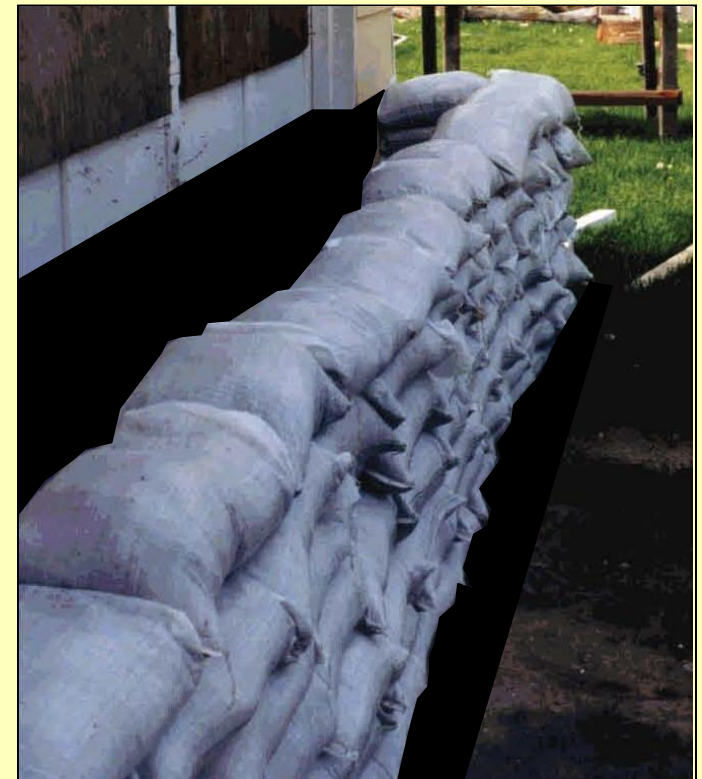
To protect a structure, tape plastic to the walls. Stack overlapping layers of sandbags on plastic and up wall against plastic.
