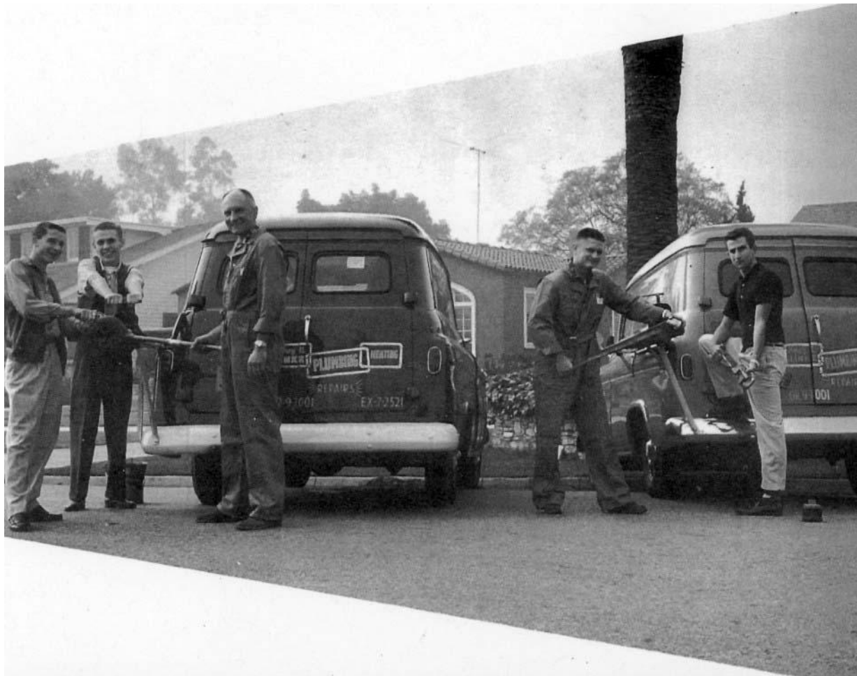
Henry H. Linke (center) ran his plumbing business in the early days from his house at 3869 Marcasel. His wife Fern was instrumental in getting the name of the street she lived on changed from West Blvd. to Marcasel Ave. The reason why the roadway was downgraded from a boulevard to an avenue would be interesting to know. The photo was taken in 1958.
