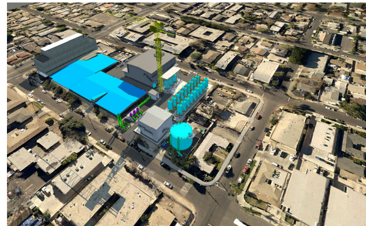
The North Hollywood Central Treatment project is a groundwater treatment facility to treat 38.2 cfs of groundwater for contamination from the Rinaldi Toluca wellfield. This project is part of Water System’s
