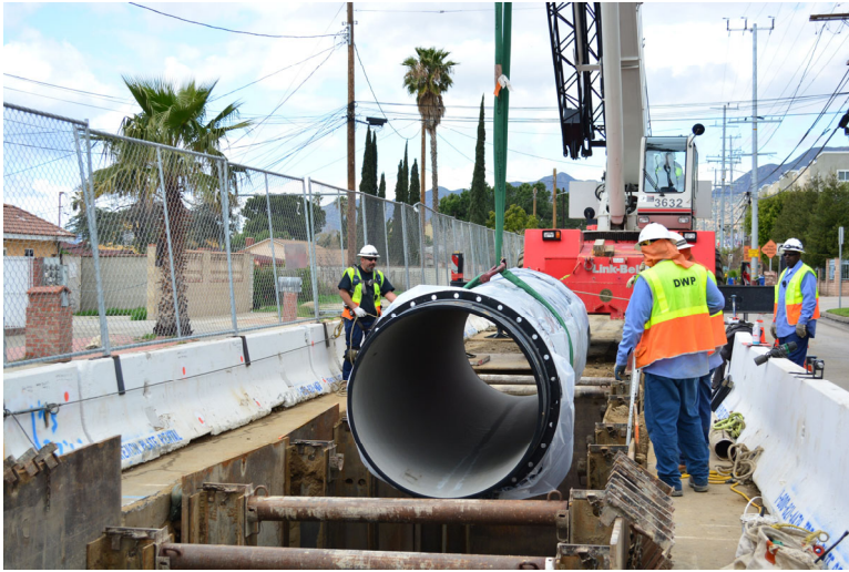
The Foothill Trunk Line Project will install 16,600 feet of 54-inch welded steel pipe and earthquake resistant ductile iron pipe using the open trench method and pipe jacking. 4,361 feet of pipe has been installed by Trunkline Construction to date.
