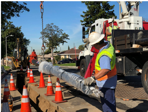
The Foothill Trunk Line Project will install 16,600 feet of 54-inch welded steel pipe and earthquake resistant ductile iron pipe using the open trench method and pipe jacking. 4,361 feet of pipe has been installed by Trunkline Construction to date.
