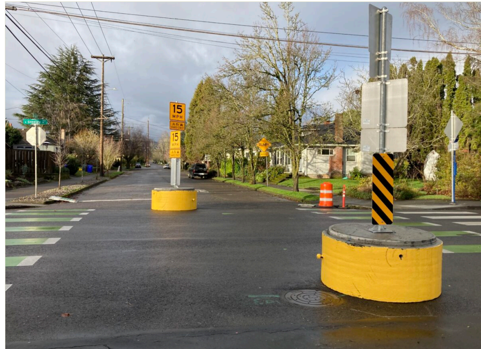
That's one serious traffic calming feature. View is looking west on Bryant across Greeley. (Photos: Seth Sokol)
