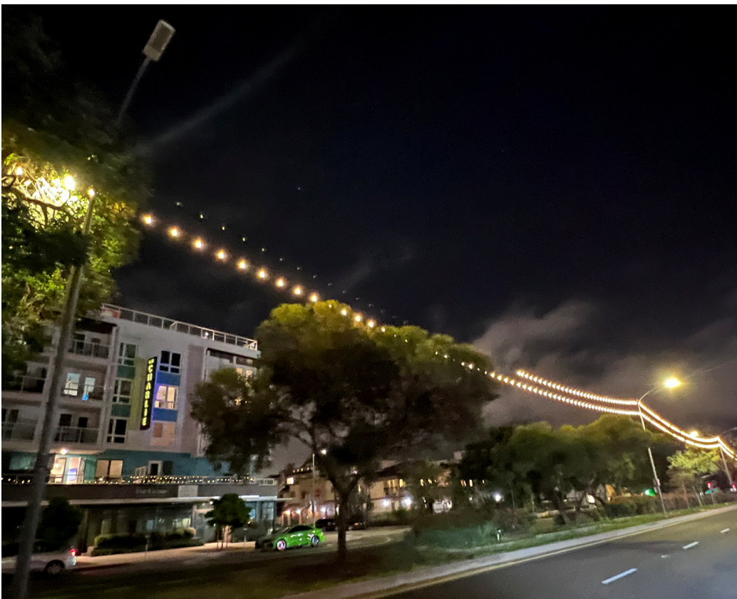
Partial lines and bulbs are out here at Venice and Centinela.
